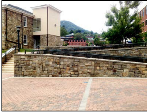
Fig 15: the handicap ramp by Chapell-Wilson Hall
